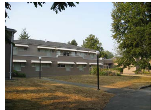
South side of building
