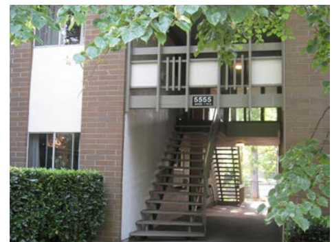
Typical building entrance
