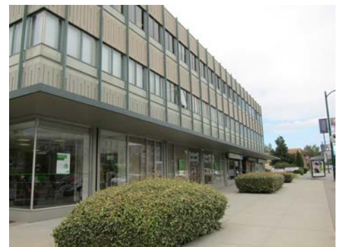
Northwest corner - retail and office space
